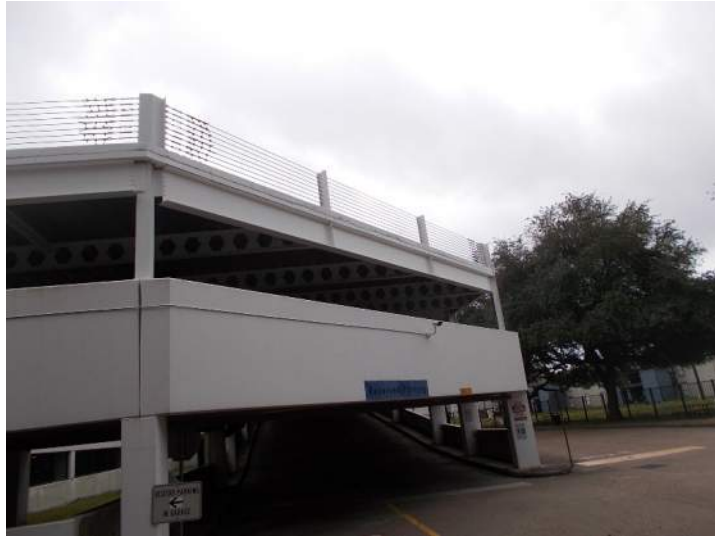
Photo 0.05 General view of southeast corner
