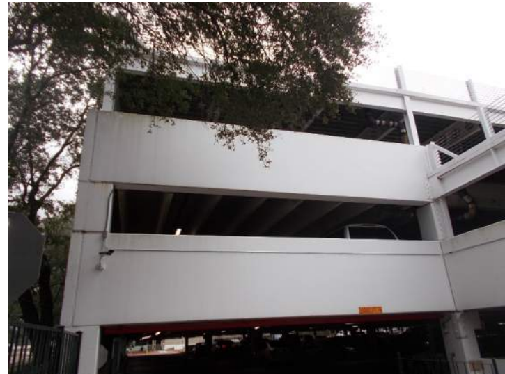
Photo 0.03 General view of south side
