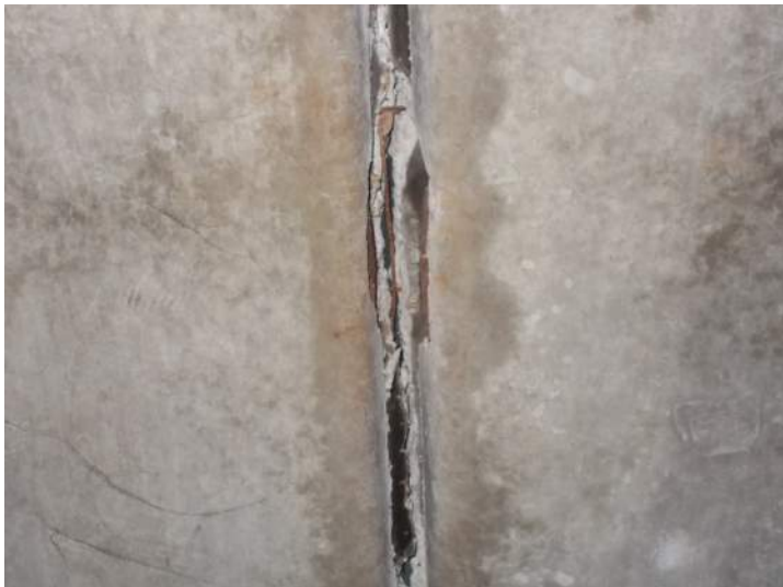
Photo 7.02 Wide joint between flanges of double tees
