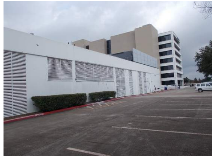
Photo 0.08 General view of east side
