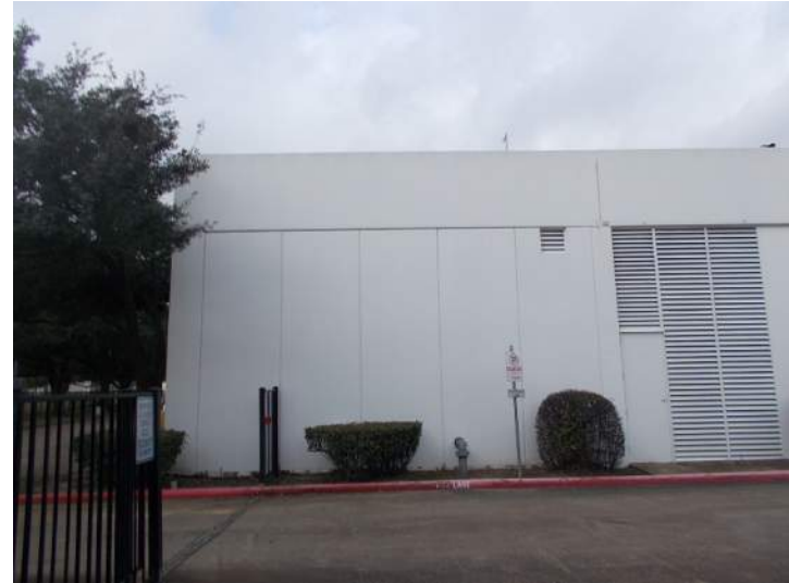
Photo 0.07 General view of east side
