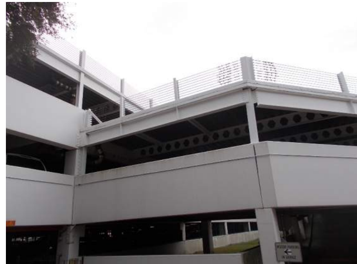
Photo 0.04 General view of southeast corner
