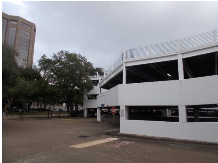
Photo 0.06 General view of south side
